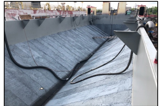
After: completed discharge hopper.
