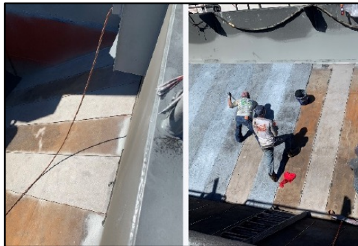
In process: screed strips welded to plate and application progressing.
