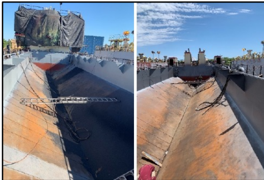
Before: dredge hopper after initial coarse blast.
